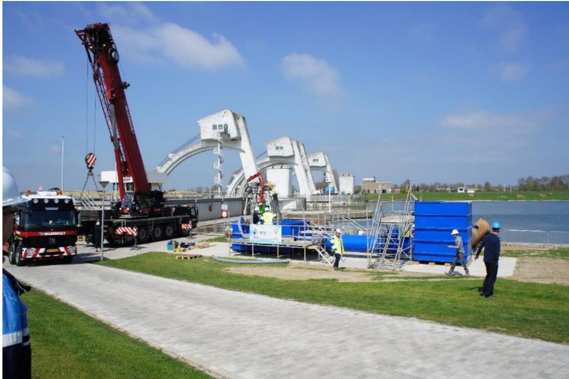
Figure 6. Building test rig on site
