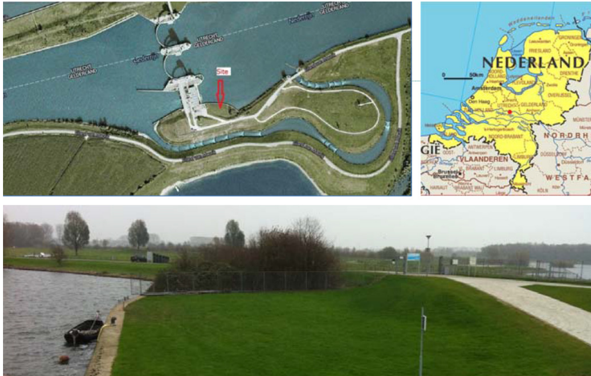
Figure 3. Right hand side (above): red dot, location of Maurik in the Netherlands. Left hand side (above): aerial view of sluices, hydro power station and fish way near Maurik. Down: view of terrain before construction of the test rig (figure courtesy of J. van Berkel)
